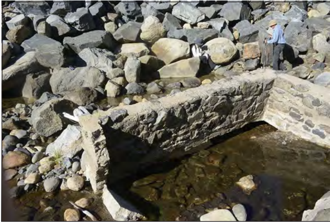
Figure 4. Remains of large water trough in South Fork American River, once used to contain saline water for medicinal purposes at Indian spring (see fig. 1 for location). Behind trough, by scientist in white shirt, are small saline ponds fed from salty-spring waters that are partly covered by blocky debris from construction activities related to widening of Highway 50, 20 m above.
